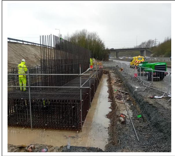
Concrete reinforcements on both sides of the A249
