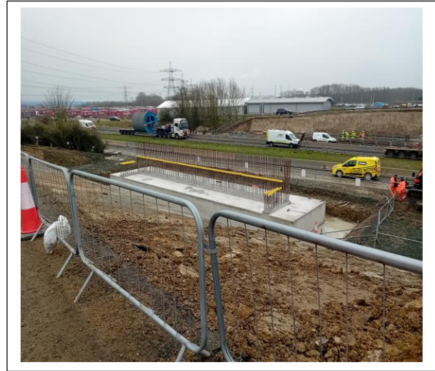
Concrete reinforcements on both sides of the A249
